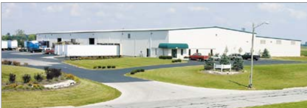
AFT is located in the Crossroads Industrial Park in Bucyrus, Ohio.
